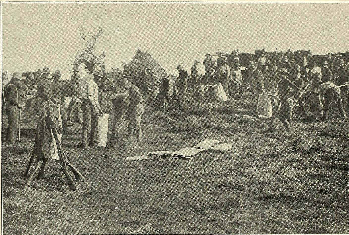
The Tenth Pennsylvanias Building Trenches at the Extreme Front.
