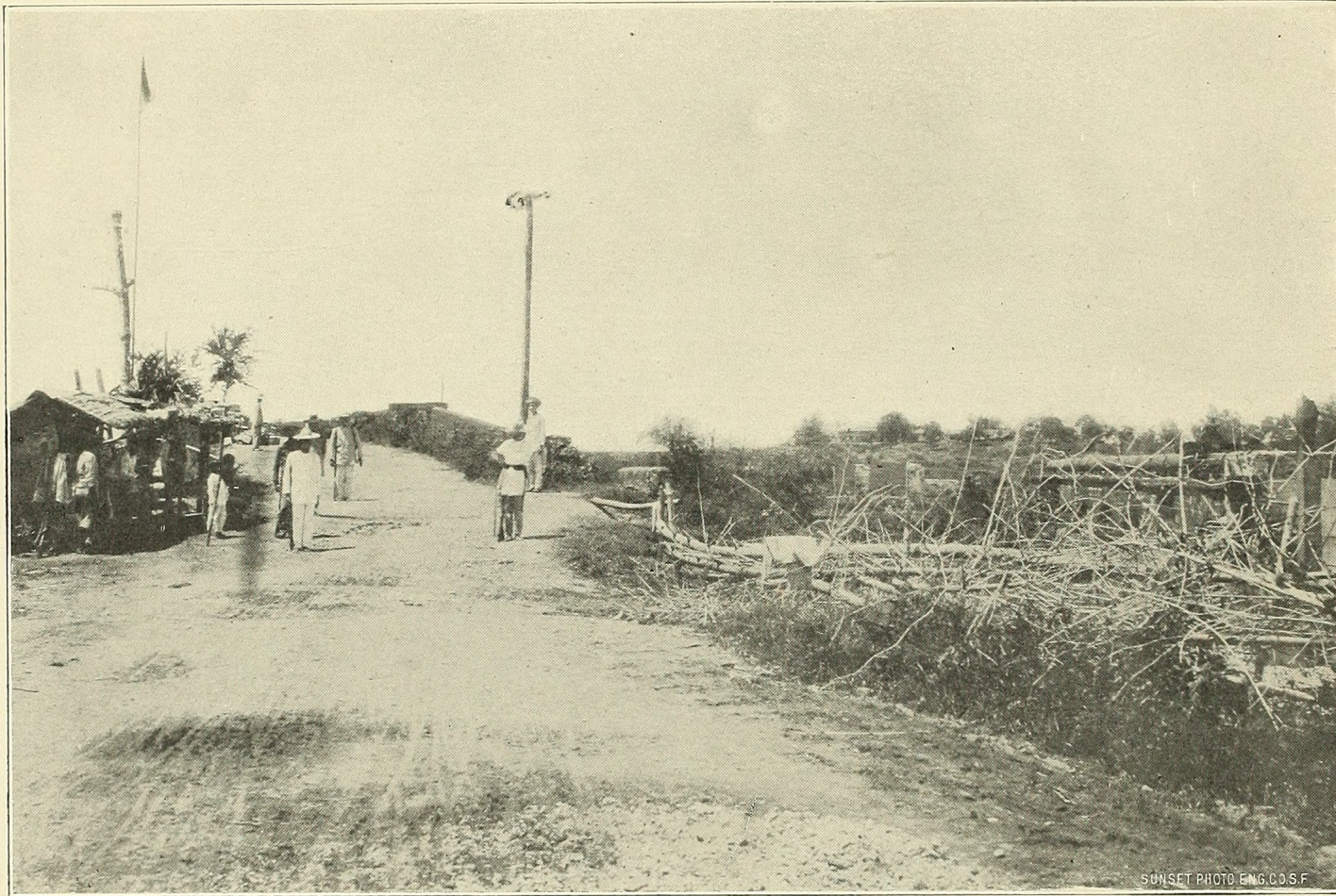
San Juan del Monte Bridge, showing Filipino Outpost, where Wm. Grayson of the First Nebraska fired the first shot of the Filipino War, February 4, 1899
